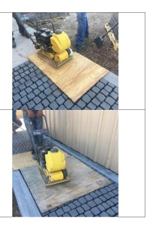
**NOTE:** <u>Do not</u> drive on or disturb the surface in any way prior to applying joint infill. Avoid walking on the surface where possible. It is easy to snag cobbles with the toe of your shoe, causing part of the mat to be unseated from the base. It is highly recommended to create a visible barrier so workers know not to walk or drive on the finished surface.
