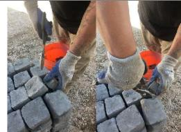
At the area of placement, have one team member lower their end of the mat into place first. Use joint spacing sticks against any curbs to achieve the correct joint width.
